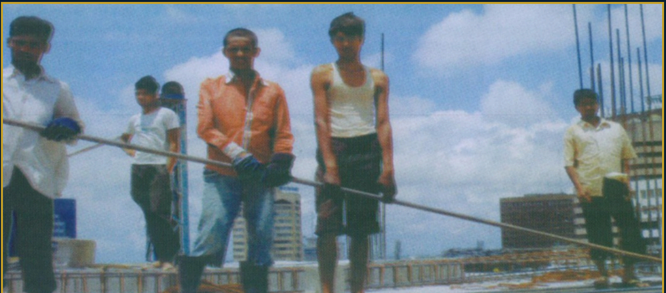
Construction site deployment
